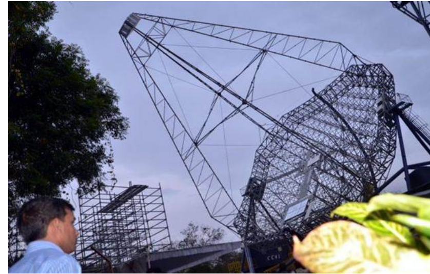
MACE - Major Atmospheric Cherenkov Experiment, Ladakh, India, 4200 m a.s.l, mirror 21 m
